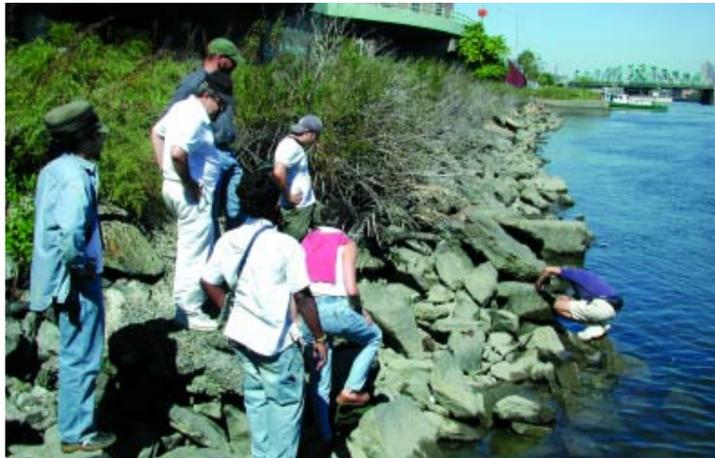
scour along the edge and river bottom; absorbs wakes and wave action; and still functions to hold back landfill that supports upland uses.
