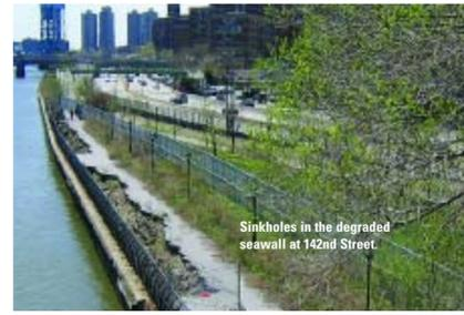
Sinkholes in the degraded seawall at 142nd Street.
